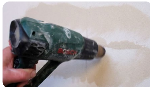
Drying the surface with a heat gun (2:00)
