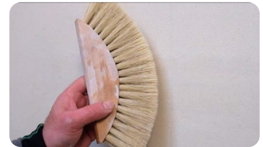
Final phase: brushing the surface (4:15)
