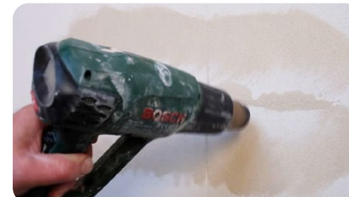
Drying the surface with a heat gun until leather dry (2:50)
