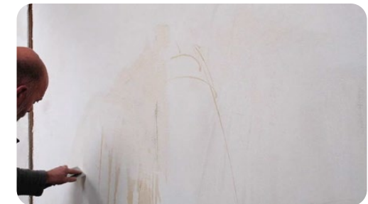
Removing most of stained CF (1:25)
