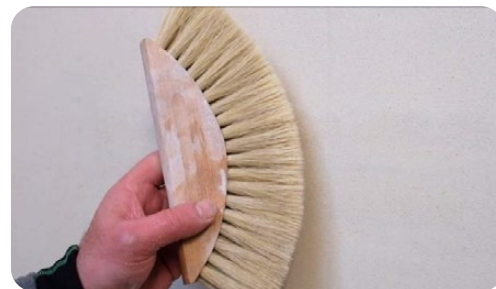
Final phase: brushing the surface (5:00)
