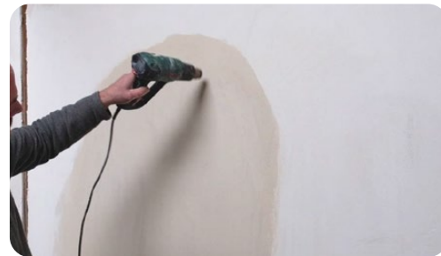
Drying the surface with a heat gun (3:30)
