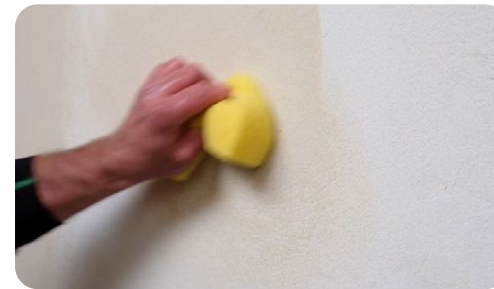
Final phase: wiping the surface (3:40)
