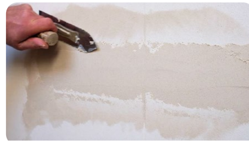
Iron edges for smooth transition (2:30)
