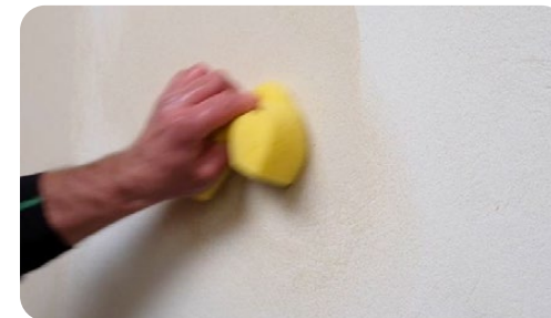
Final phase: wiping the surface (4:00)
