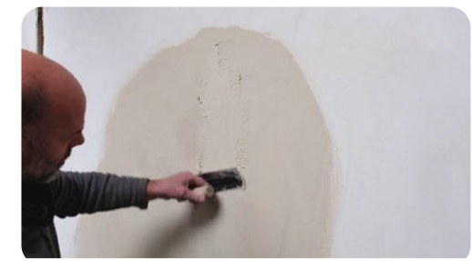
Applying the CF (2:05)
