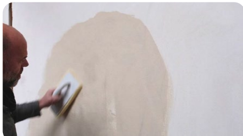
Wiping repaired surface (2:40)
